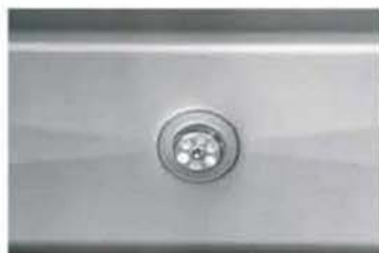
≡ Photo 15: centralised drain
